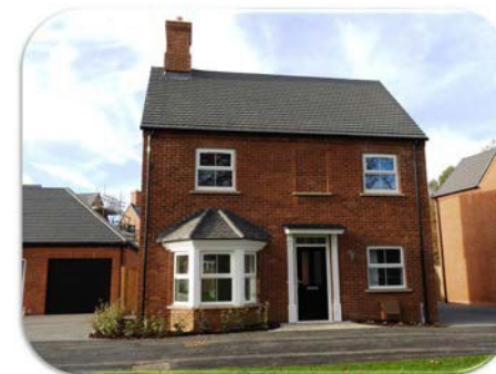
New homes on the former RAF Upwood clinic site, Bury
